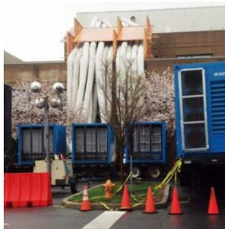
*The rental ventilation equipment needed to substitute for the ruined fan and motor.*
