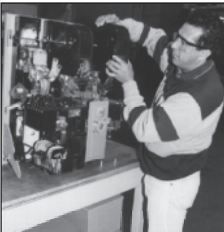
Circuit breaker being reassembled after upgrading at Wharton Center.
