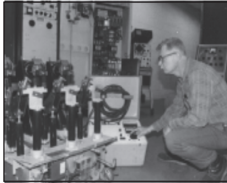
Circuit breaker being high potential tested in our laboratory.
