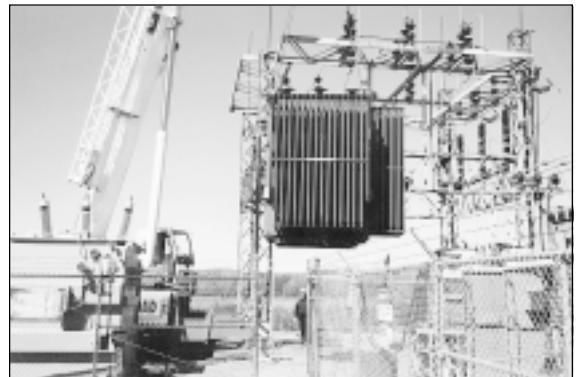
Old unit being removed
