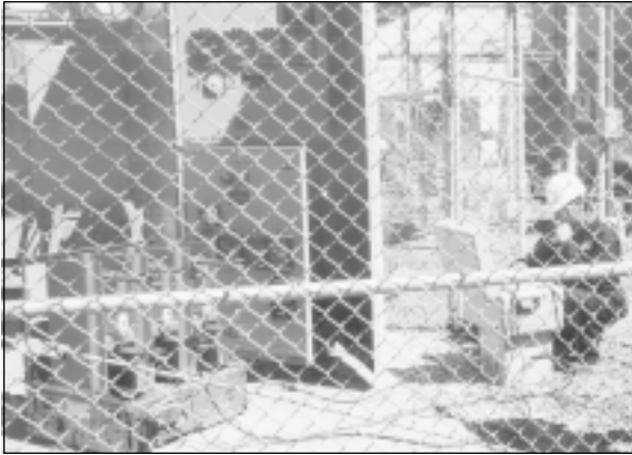
Testing the breaker
