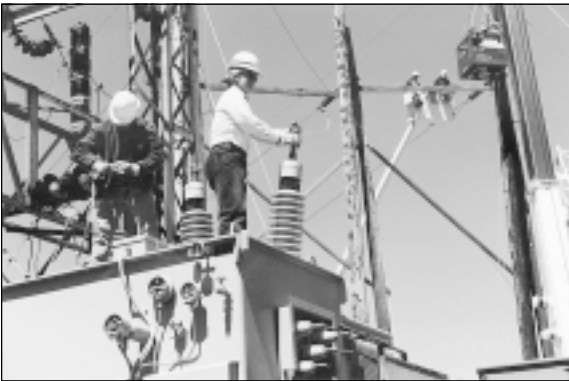
Project manager reviews details
