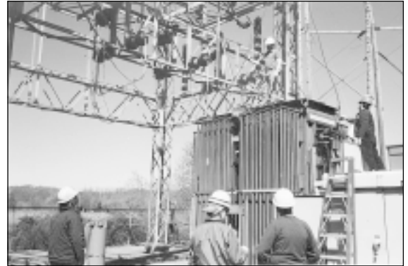
Old unit being staged for removal
