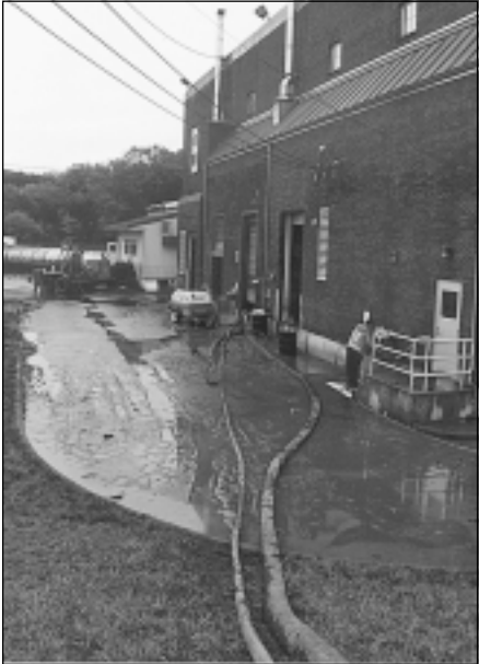
Parking lots covered with thick mud were witness to the enormity of the damage. Here even as our crews were working, pump out went on around the clock.
