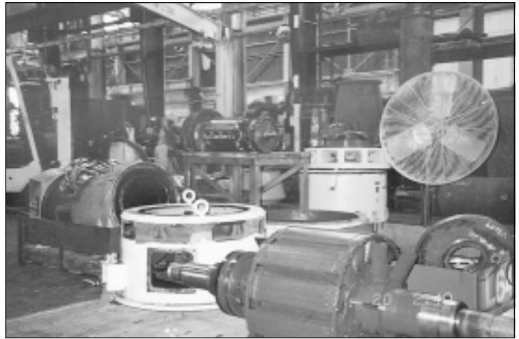
Keeping up with the field crews our 3 repair facilities were up to the task. Wharton, Linden and NYC kept the pace until the emergency was over. Here, components are staged prior to assembly
