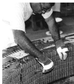
After the winding removal, the disassembly of the damaged stator laminations begins.
