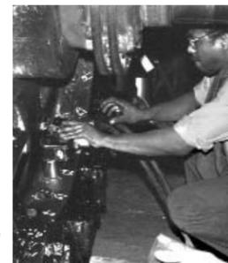
Mechanic and supervisor tighten rotor pole bolts using hydraulic calibrated torque wrench.
