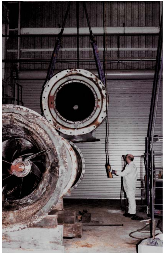
Above: You see the size of the pump and its sections. The right equipment, a 25 ton crane, and correct rigging makes the disassembly of the giant pump seem like childs play..
