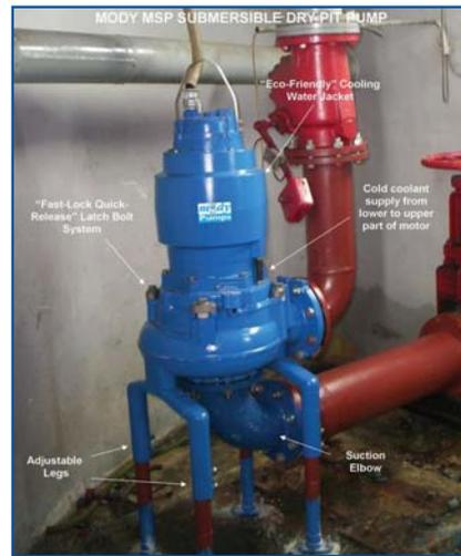
Figure 3. Retrofit installation of the Mody MSP submersible dry pit pump.
