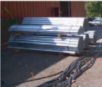
*6,000 feet of conduit was needed for the cables to replace main buss running through the building. Obtaining a replacement buss would not have been time effective.*
