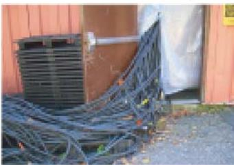
*An extensive web of cables from the generator trailers had to be organized and channeled to the correct stations to re-energize the facility*
