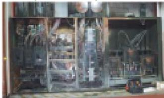
*The extent and heat of the fire is evident from the damage in the switchgear units. However, note the plastic mirrors above the cabinets. Electrical fires can be very unusual in how they do their damage.*
