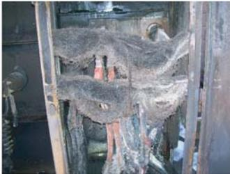
*Remnants of the transformer that ruptured and sent burning oil into the switchgear area.*
