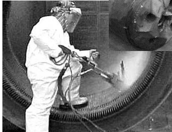
final machining. Simultaneously, Longo technicians geared up to wind the stator and repair the damage to the lower end of the motor. Teaming up with our supplier/partner TECO/Westinghouse, we were able to get several critical parts fabricated in 72 hours. Work proceeded around the clock through the weekend.
