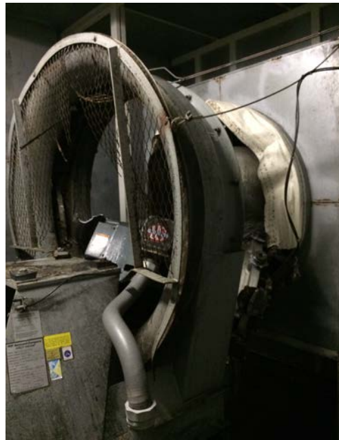
These two photos show the aftermath of the fan that exploded. On the far right you can see where the 1700 lb. motor was torn right off its mountings! Definitely validates stories of fan blades slicing through cinder block walls.
