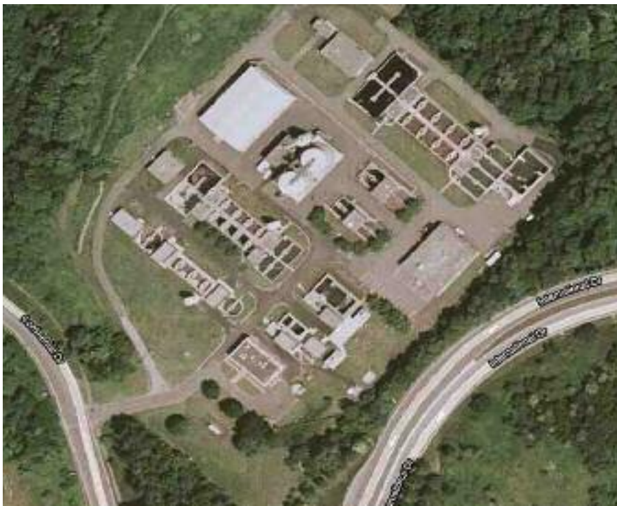
The project required Longo to replace 55 VFD's that control all the various pumps throughout the complex. The units varied in size from 10 hp to 20 hp.
