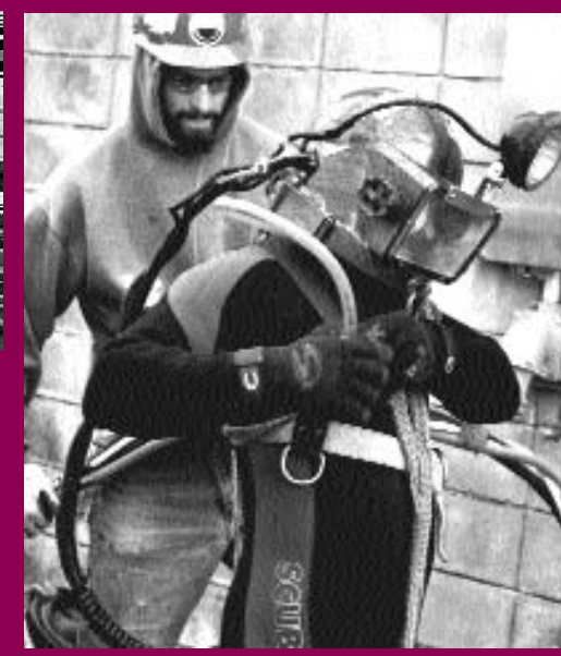
Divers were critical for the extraction, positioning and aligning the jack beneath the pump, adding the needed pressure to break the pump loose from the encrusted casing.
