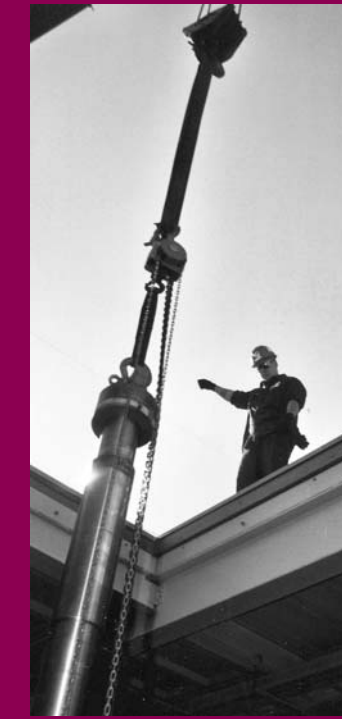
The reconditioned pump was stopped just above the casing rim. It was suspended while the special adapter was removed from the pump shaft so the main shaft from the motor to the pump could be lowered into position.
